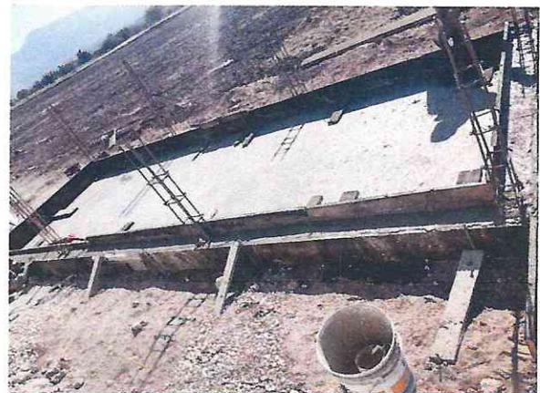
FIRME DE CONCRETO HIDRAULICO HECHO EN OBRA DE  $f'c = 200 \text{ KG/CM}^2$  DE 10 CM, CIMBRA DE CONTACTO ACABADO COMUN EN CADENAS Y CASTILLOS, ACERO DE REFUERZO EN ESTRUCTURA CON ALAMBRO # 2 y # 3, CONCRETO HIDRAULICO HECHO EN OBRA  $f'c = 200 \text{ KG/CM}^2$  EN ESTRUCTURA.
